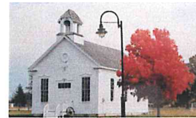
5080 Wildcat Road (across from the Dorsey House)
